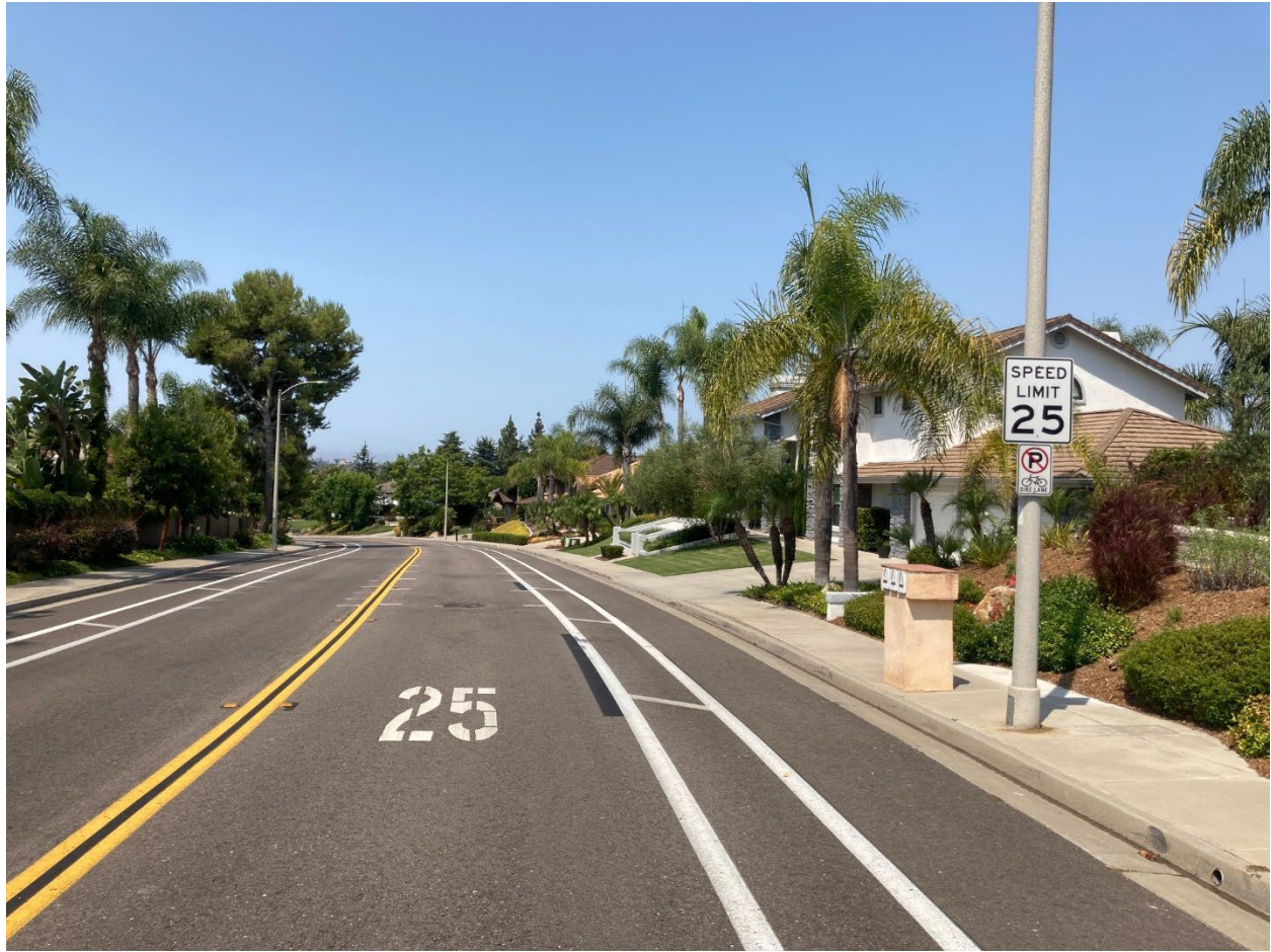
Phase I – Speed Limit Sign and Marking and Lane Narrowing
