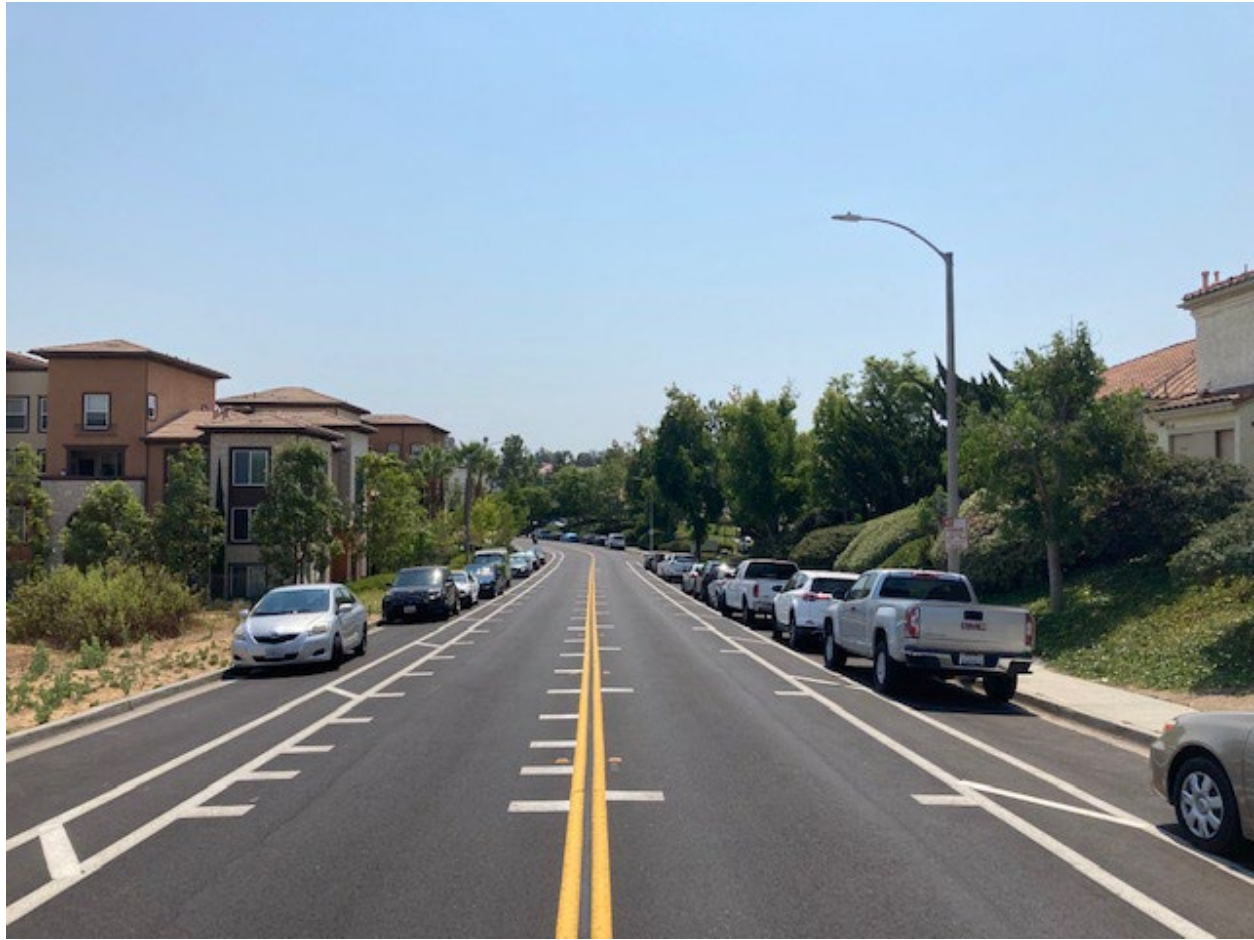
Phase I – Speed Reduction Markings and Parking Lane Buffer
